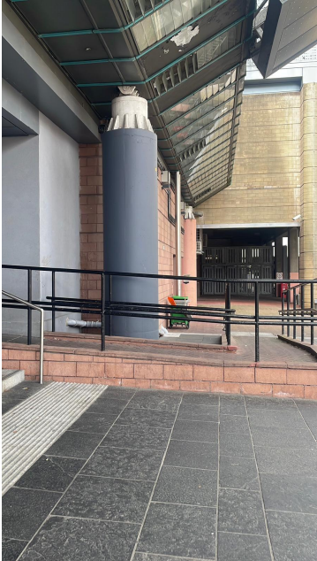
There are 4 steps into the entrance and a wheelchair ramp
